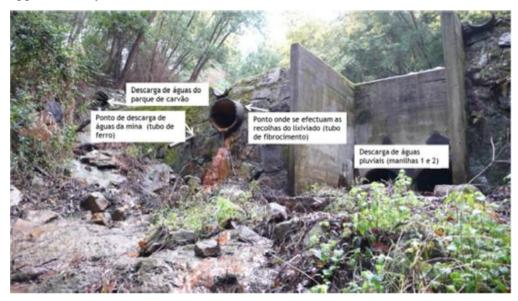
Figure 7: Aspect of water collection system on the study area
