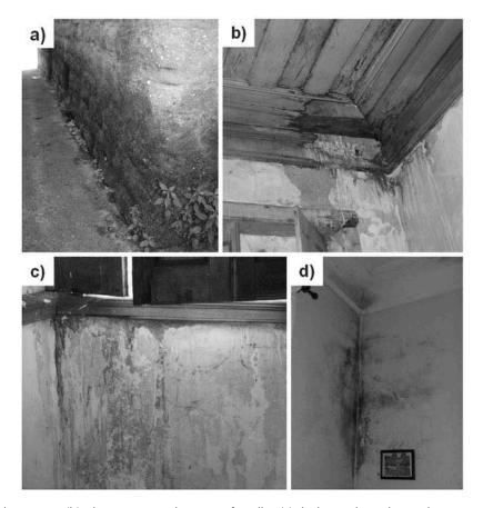
Figure 8. (a) Rising dampness; (b) dampness at the top of walls; (c) leakage through window openings; and (d) surface condensation.
