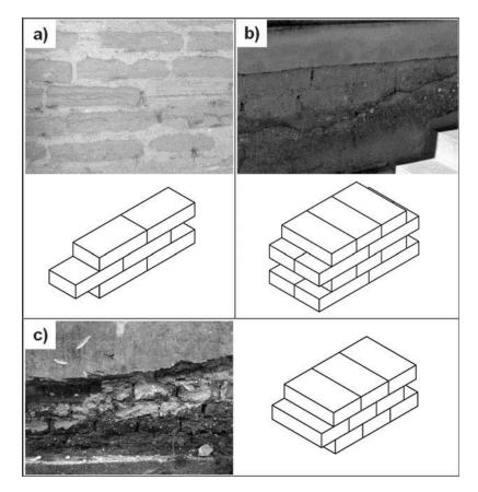
Figure 3. Types of adobe masonry bond: (a) stretcher bond; (b) English bond; and (c) header bond.
