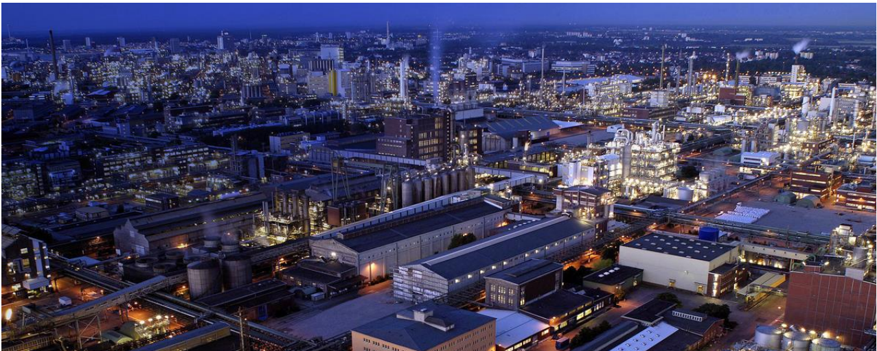
Fig. 1 - BASF Headquarters Ludwigshafen am Rhein, Germany.
