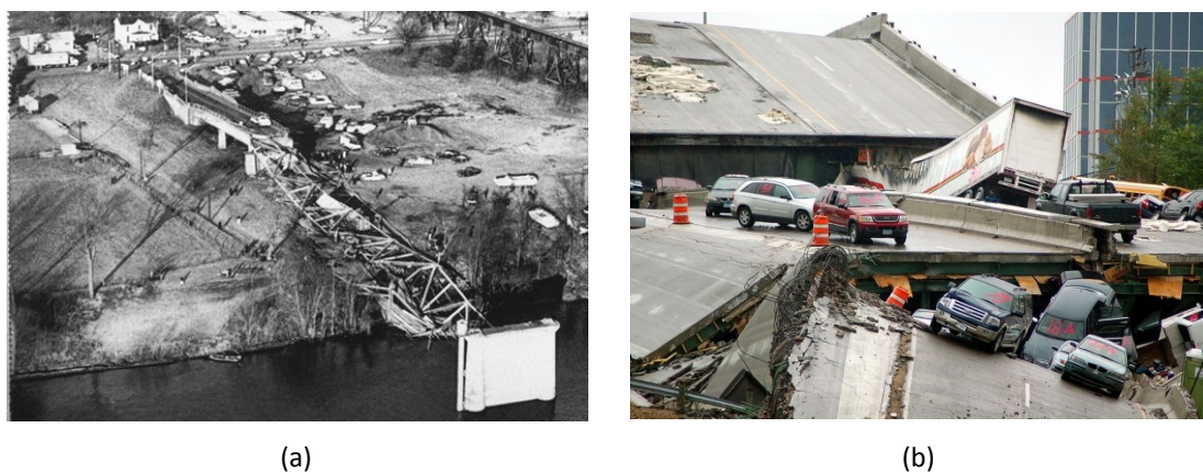
Figure 1.1 – Collapses of: (a) the Silver Bridge, at Point Pleasant, West Virginia, in the USA; and (b) the interstate highway bridge I-35W over the Mississippi River in Minneapolis, Minnesota, in the USA.
