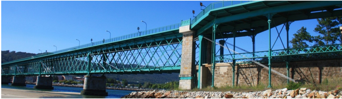
Figure 3.3 – View of the Eiffel Bridge highlighting the external prestressing system.
