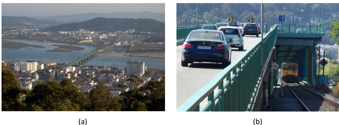
Figure 3.1 – Eiffel Bridge: (a) general view; and (b) southern viaduct.
