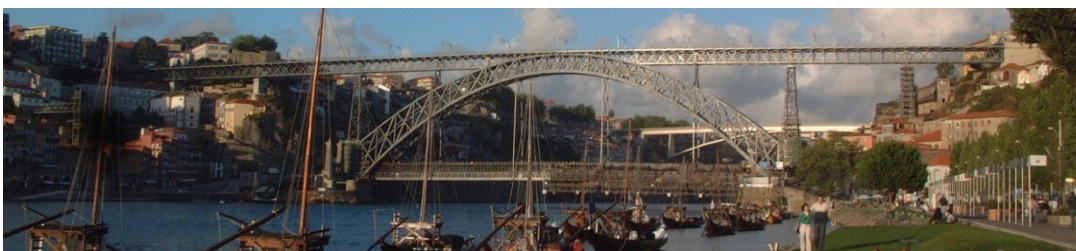
Figure 8.1 – General view of the Luiz I Bridge (North (Porto) on the left and South (Gaia) on the right).
