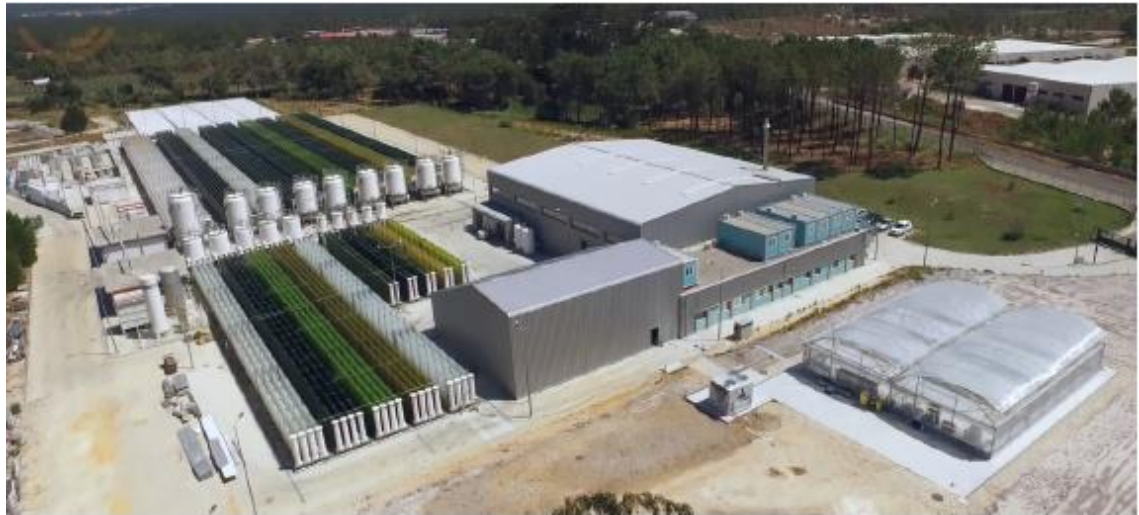
Figure 3 – ALGAFARM facilities (from: Silva et al. 2017).
