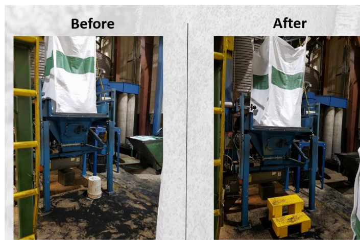
Figure 44 - Loading operations improvement measure
