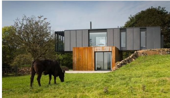
Figura 2.27 – Grillagh Water House [35]
