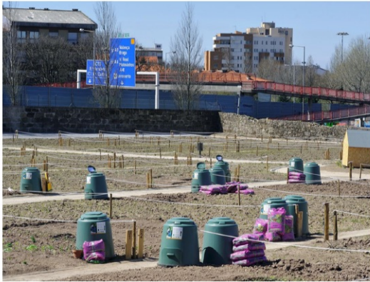
the park under construction
