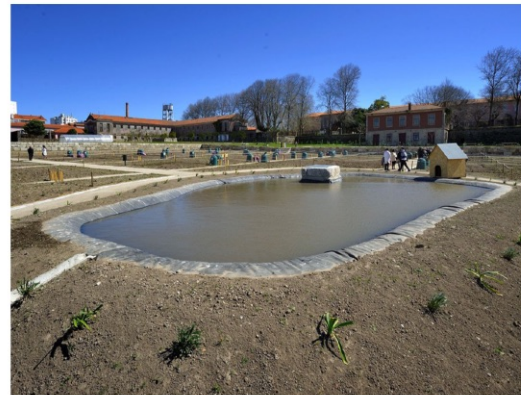
rain water storage
