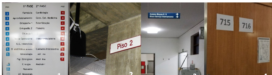
Figure 1 – 1&2. Lack of maintenance of the directory and signage obstructed by the Television (Hospital de Santa Luzia - Viana do Castelo)/3. Signage with small letters (Hospital Infante D. Pedro - Aveiro)/ 4. Paper sheets taped on doors to overcome lack of signage (Hospital de Santo António – Porto)
