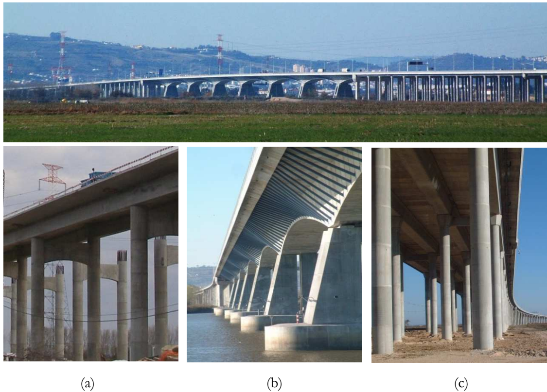
Figure 6.17 – An overview of the Lezíria Bridge and each of the three structures: (a) northern approach viaduct; (b) main bridge; (c) southern approach viaduct.
