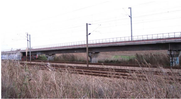
Figure 7.4 – First three spans of the north ramp.
