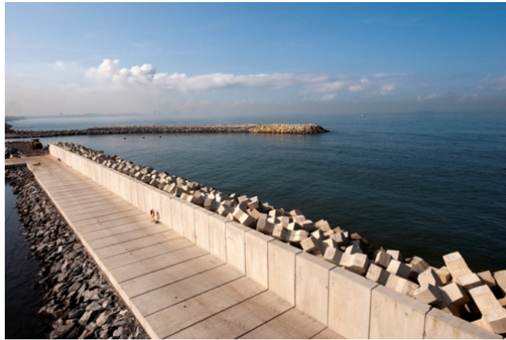
Figure 4.1 - Breakwaters Dikkowita, Sri Lanka.
