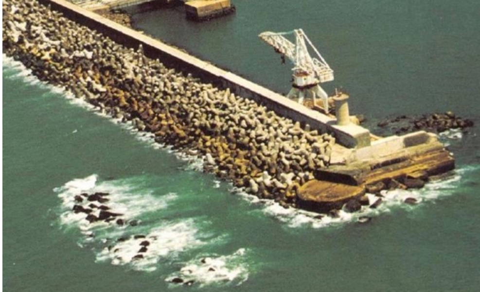
Figure 4.11 - North breakwater's head with submerged breakwater, Port of Leixões, (Veloso – Gomes et al. , 2013).
