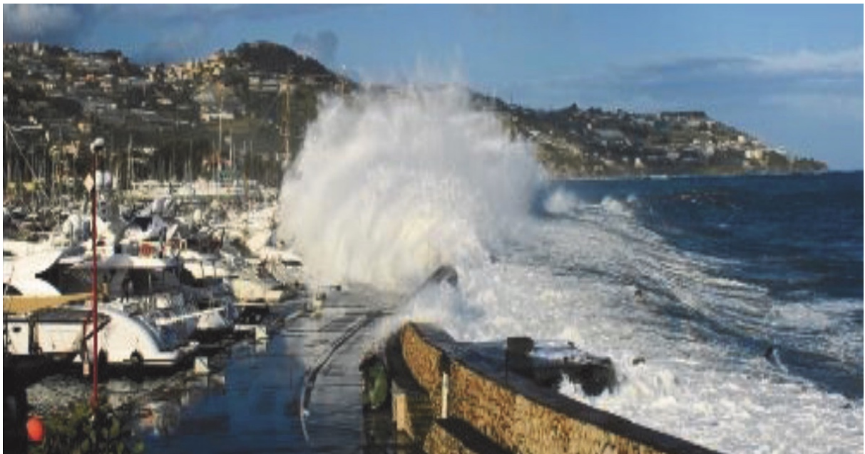
Figure 3.1 - Wave overtopping at the marina of San Remo, Italy, damaging small boats (Eurotop II, 2016).
